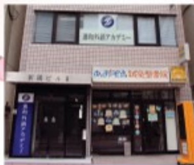
Building 2 (2F - 4F)
